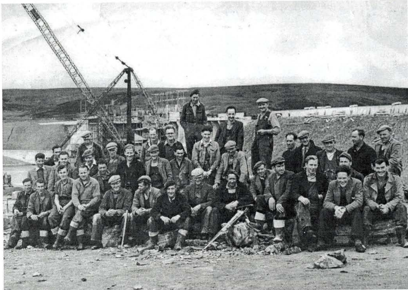
Working on the dam at Lairg, recognise any faces?
